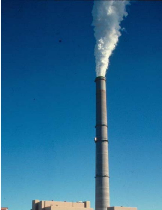
Wet flue gas desulphurization (FGD) stack
